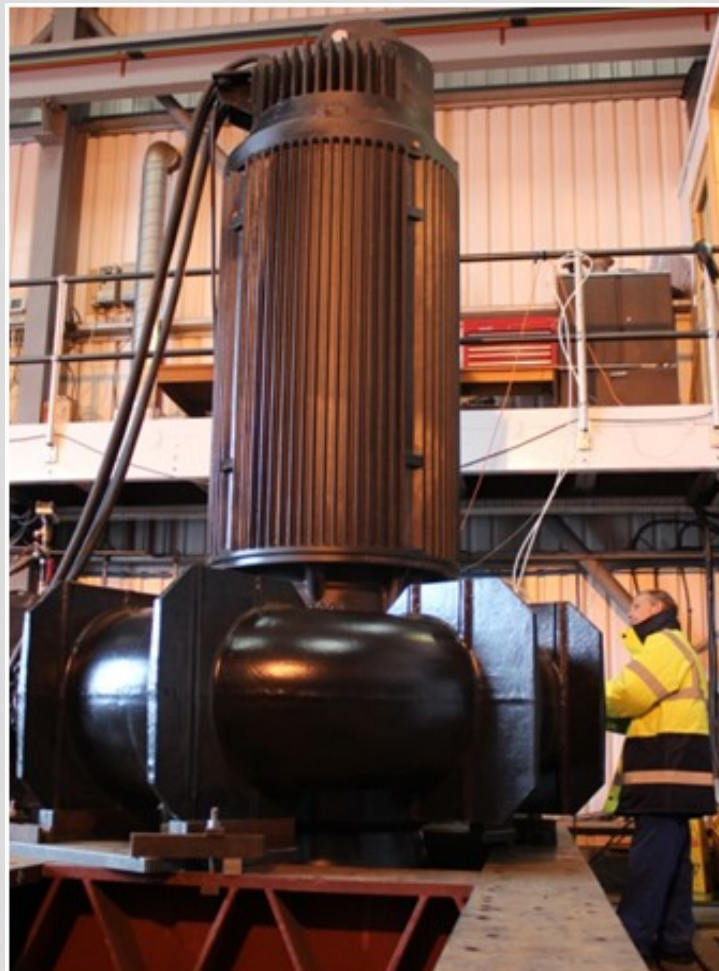
Bedford Pumps replacement which will utilise the existing concrete plinths
