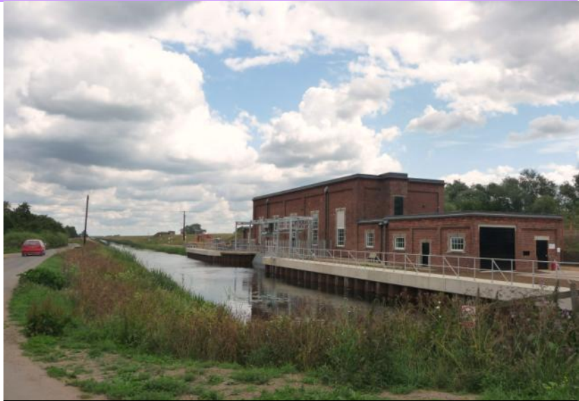
Welches Dam Pumping Station in the Cambridgeshire Fens
