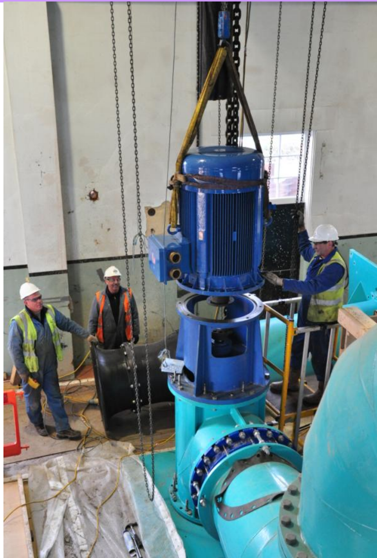
Installing the pumps at Welches Dam
