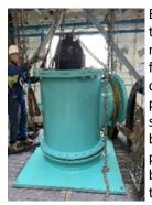
Bedford Pumps scope of supply included the two axial flow submersible pumps, a multi-section canister with a cruciform inlet, fish friendly siphon breaker valves, a pump condition monitor, as well as removal of the previous pump, installation and commissioning. The restricted height on site bought its own challenges to the installation process but Bedford Pumps overcame this by installing and removing the pumps in the top section of the canister.
