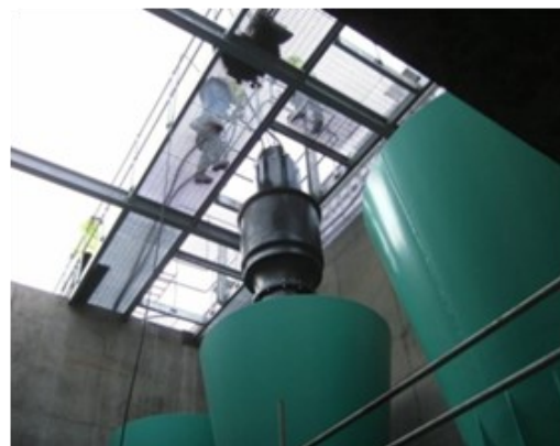
Fig 3. Pump installation at Minworth
