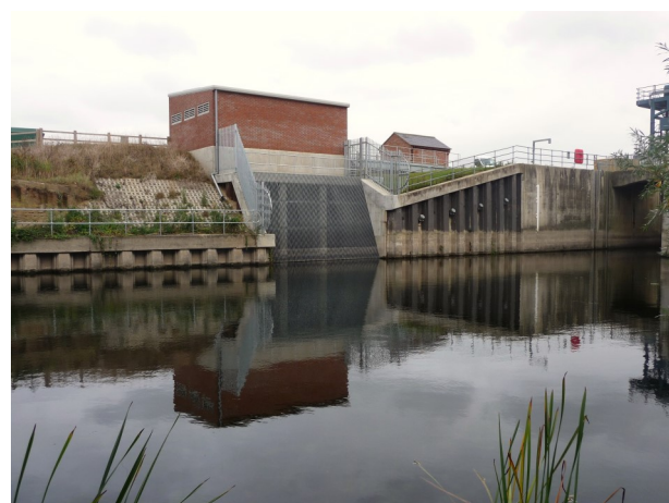
Welmore Lakes Transfer Pumping Station
