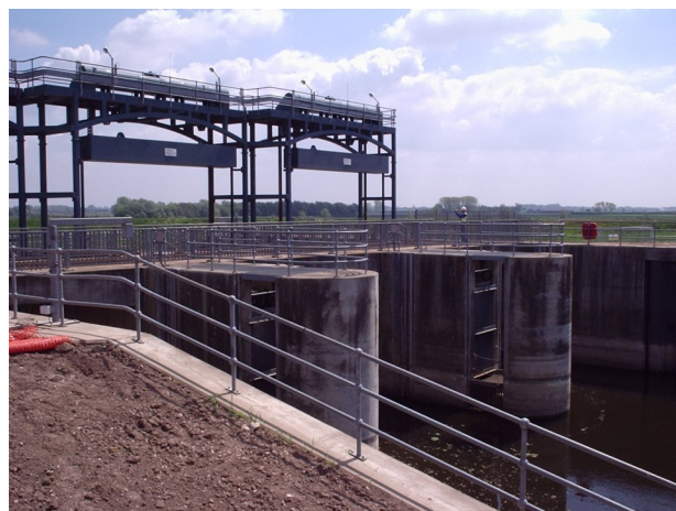
Welmore Lake Sluice
